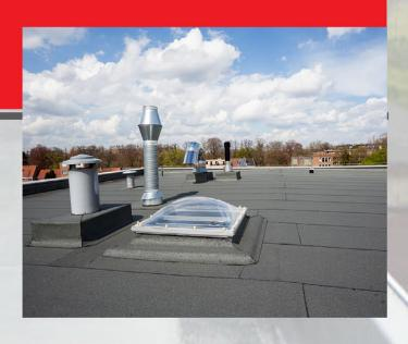
The reinforced three layer insulated membrane is resistant to impact and tearing, whilst being flexile to climatic extremes and structural movement giving complete peace of mind over a 40 year life expectancy.
